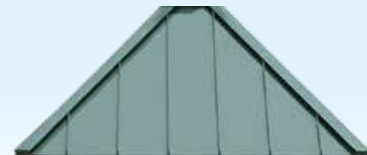
Standing Seam Metal Roof
